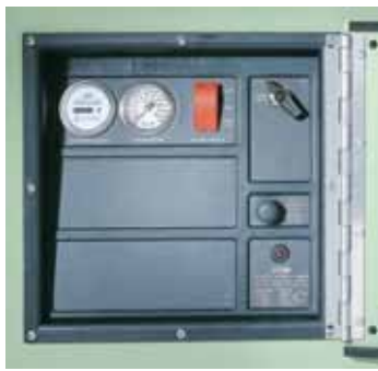
Curbside Instrument Panel With (SSAM) Shutdown System & Annunciation Module.
